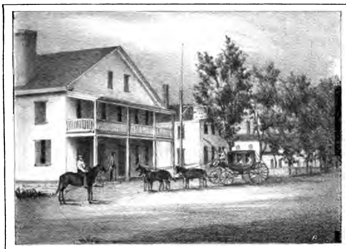
TURNER'S HOTEL, UPPER END OF N VILLAGE
