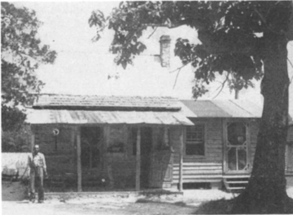
FIG. 15. Log cabin built by veteran of Mexican War. The kitchen-dining room at right has been added at a later date.
