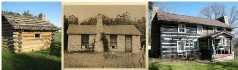
Types of permanent homesteads then popular – log cabin, stone (an old picture of the home of Mohegan medicine woman Tantaquidgeon), and cut log with clay, mud or plaster filler
